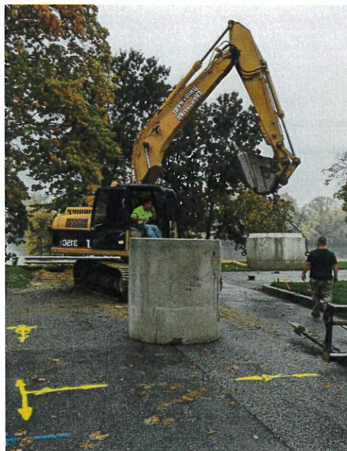
Setting deep sump catchbasins with pretreatment device and diversion manholes. (October, 2022)
