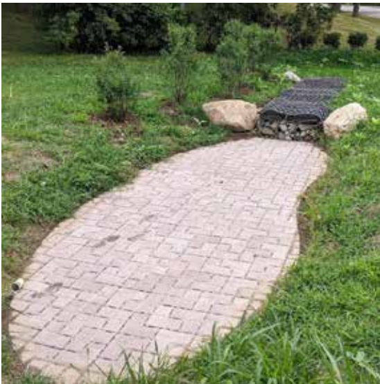
What appear to be patios are actually pathways of permeable pavement that direct stormwater to a containment area to remove sediment. The water then travels on to natural filtration zones to decontaminate the roadway runoff while it seeps into the water table.
