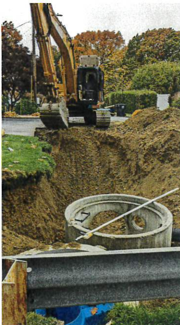
Setting deep sump catchbasins with pretreatment device and diversion manholes. (October, 2022)
