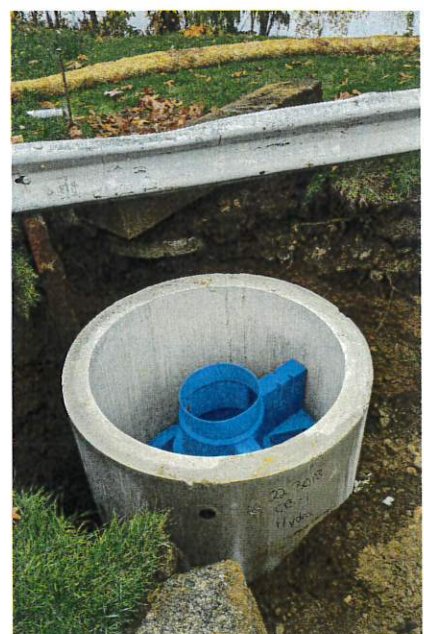
Setting deep sump catchbasins with pretreatment device and diversion manholes. (October, 2022)
